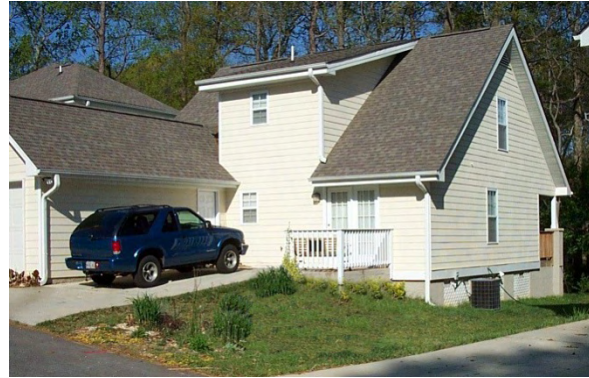
Figure 5: On steep terrain, a zero-step entrance may be more feasible at the back or side entrance.
